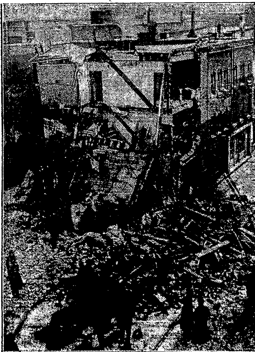
Here is an example of capitalist housing—this is all that remained of a four-story tenement in Buffalo, N. Y., in which five persons were killed, after a fire. There are thousands of fire-traps like this throughout the United States. Housing represents one of the major failures of the Roosevelt administration.
